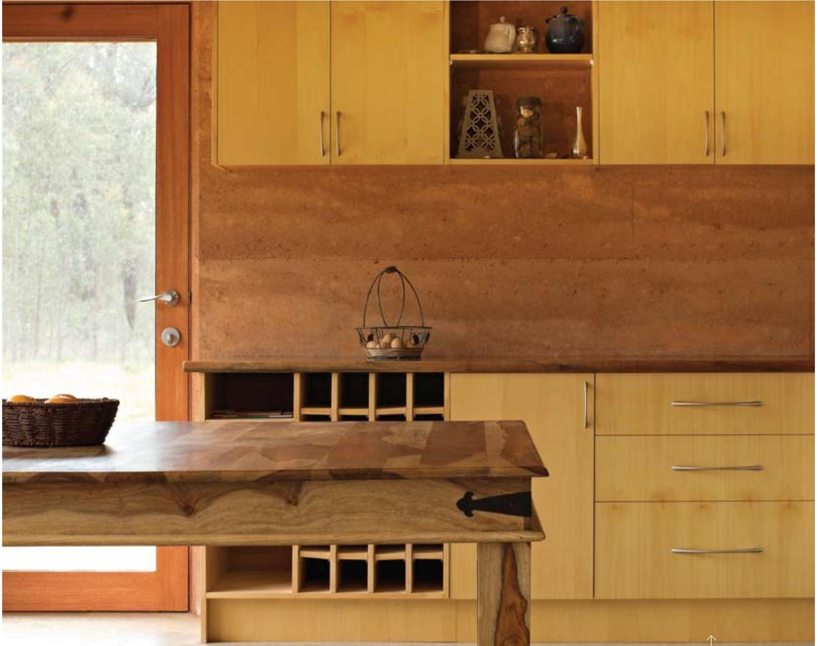
Using locally-sourced and sustainably-harvested materials to reduce the embodied energy of the house was important to the Eagles. **The stairs, window frames and hallway beams are made from local hardwood.** The kitchen cupboards are made of hoop pine harvested from sustainable plantations. The earth for the walls was quarried from a site within 25 kilometres of the house. A structural pillar in the living area was salvaged from a bridge in Howlong and still bears the marks of old bolt holes.
